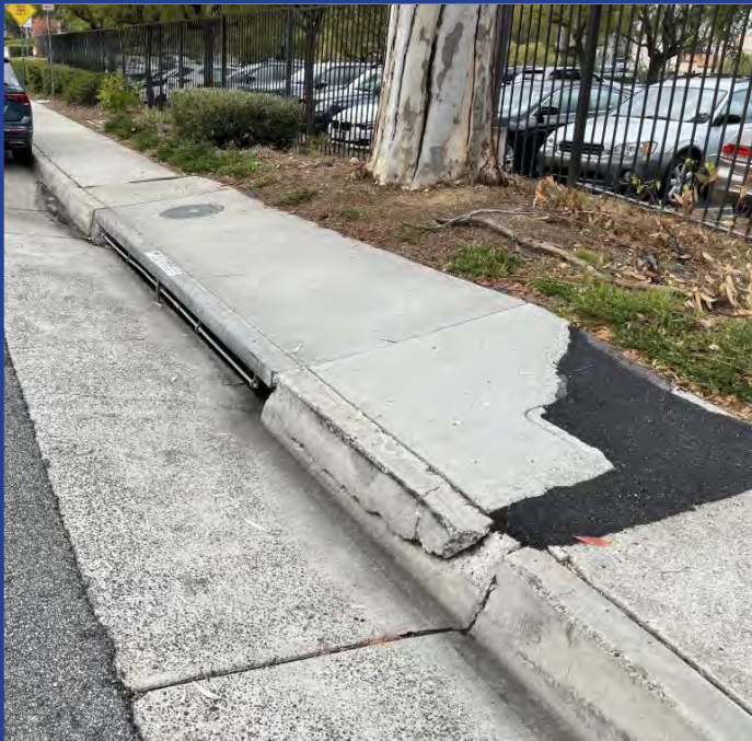
DAMAGED SIDEWALK AND CATCH BASIN
