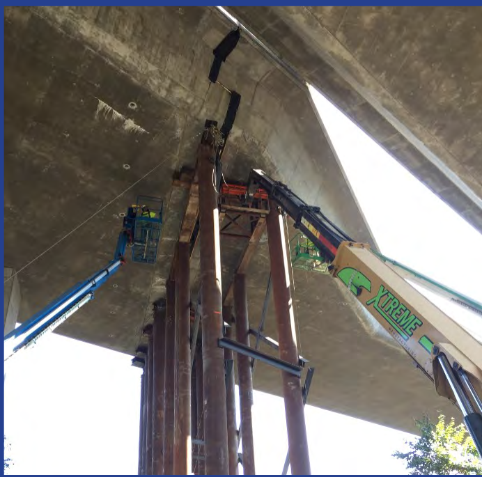
BRIDGE HINGE REPAIR
