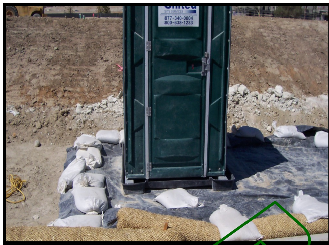
Spill containment for portable toilets
