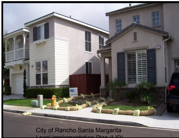
Sandbags and straw fiber rolls for runoff, erosion and sediment control
