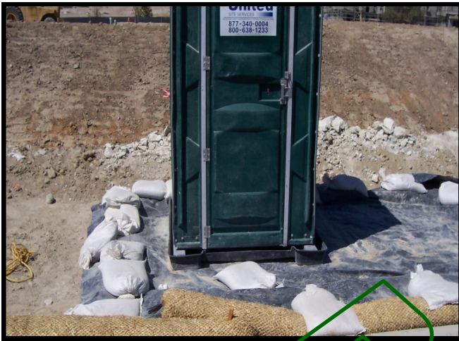
Spill containment for portable toilets
